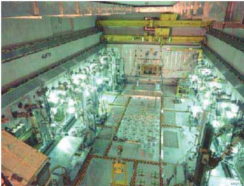
Hot fuel examination facility
