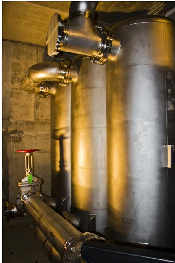
**Fig. 2.4 –  $^{16}\text{N}$  Delay Tanks in shielding vault**
