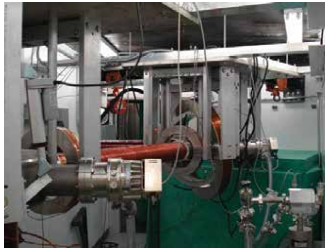
Positron beam cave containing magnetic switchyards and transport solenoids, located in the PULSTAR reactor facility on the NC State North Campus in Raleigh, NC.
