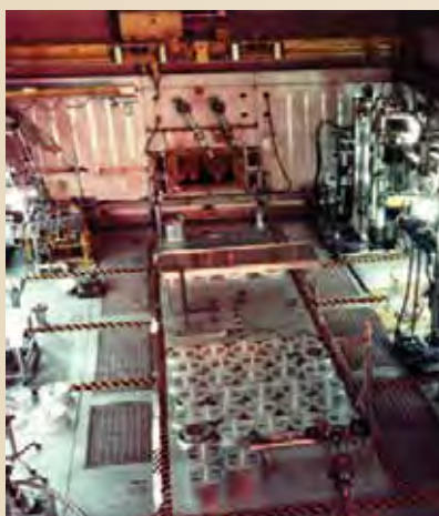
Hot Fuel Examination Facility, located at the Materials and Fuels Complex at DOE's INL Site in Idaho.
