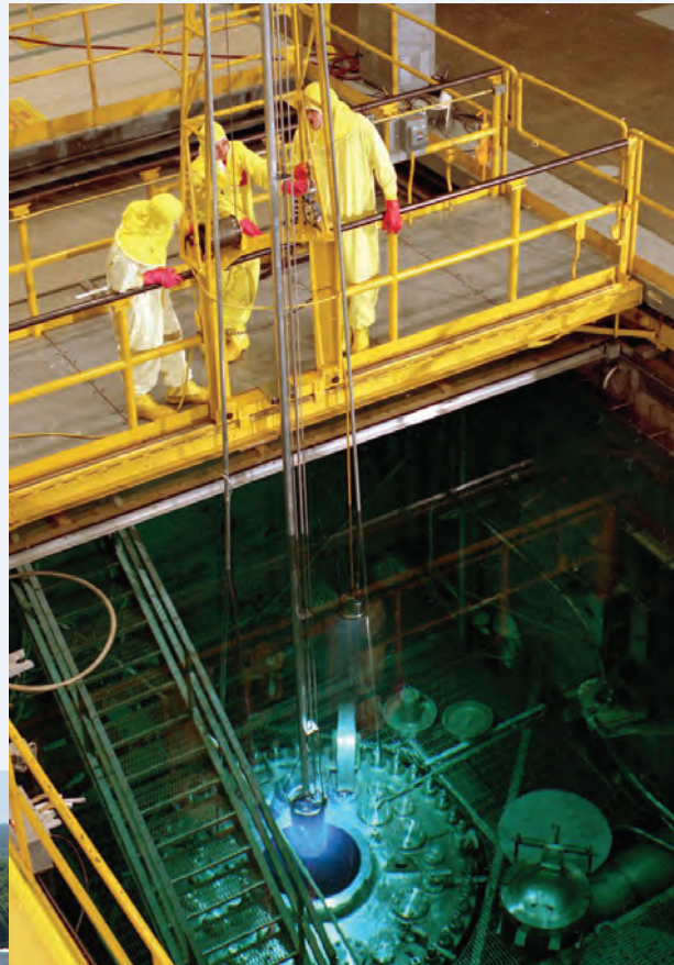
HFIR removing inner fuel element.
