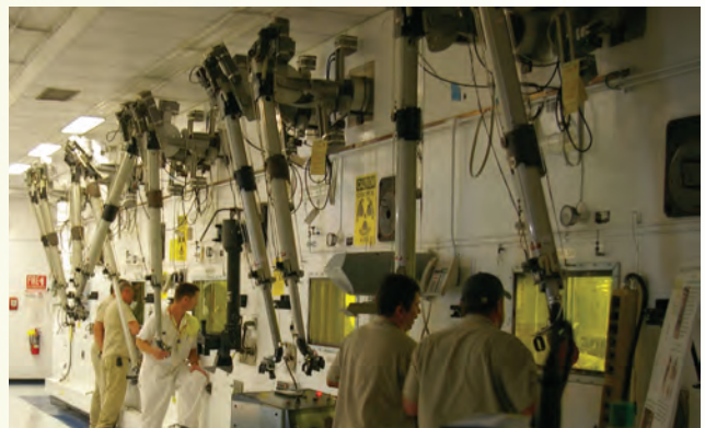
North hot cell.
