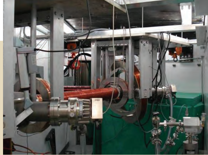
Positron beam cave containing magnetic switchyards and transport solenoids, located in the PULSTAR reactor facility on the NC State North Campus in Raleigh, N.C.
